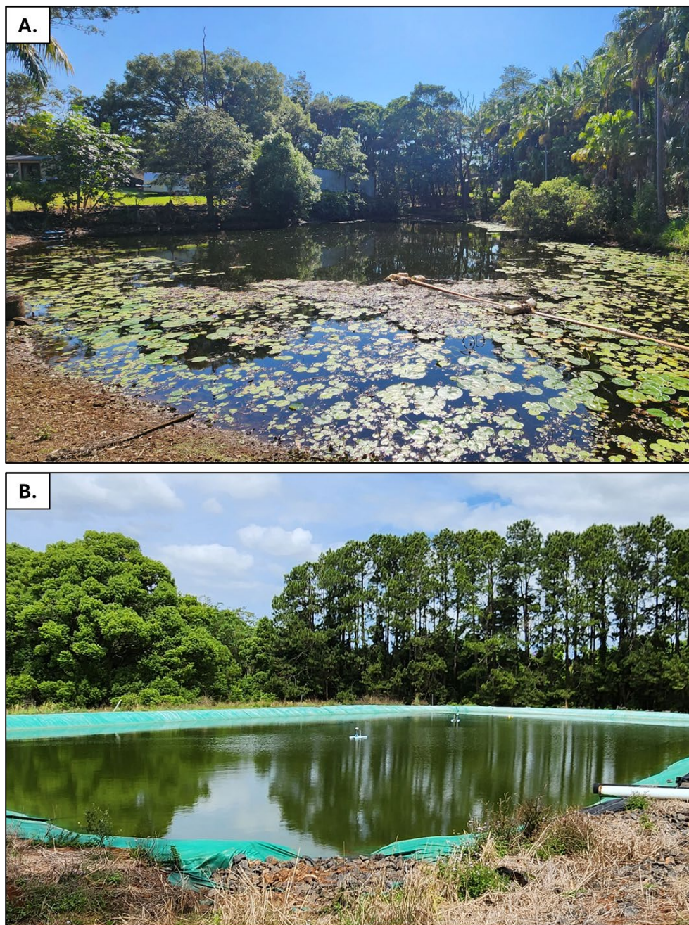
Figure 25. Example of A) unlined and B) lined water storages at production nurseries. Unlined storages lose some water to infiltration but have greater potential to support vegetation that will help to mitigate storm and flood impacts and provide wetland habitat with flow-on benefits to water quality. Lined storages lose less water to infiltration but support minimal vegetation and usually have limited wetland ecosystem benefits.
