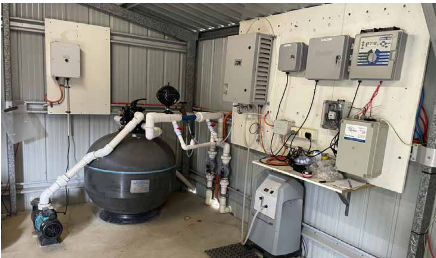
Image 2. Scott Tubes, Peats Ridge NSW – shows an ozone disinfection system, the dam water is filtered then treated with Ozone to achieve the required residual (1.4PPM) for a minimum contact time of 16 minutes.
